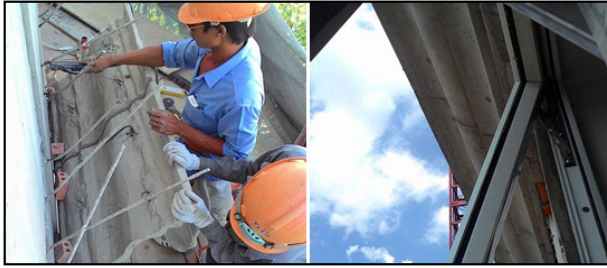
Figure 11. The installation of panels at the construction site
