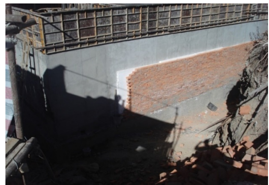
Figure 15. Foundation wall with applied hydro and heat insulation
