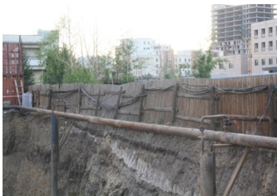
Figure 13. Water drainage system of Embassy tower: vertical and horizontal pipes
