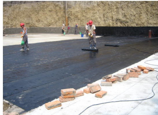
Figure 14. Application of hydro-insulation on concrete bed
