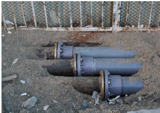
Figure 12. Water drainage system of Embassy tower: pipes for transferring water to central sewage system
