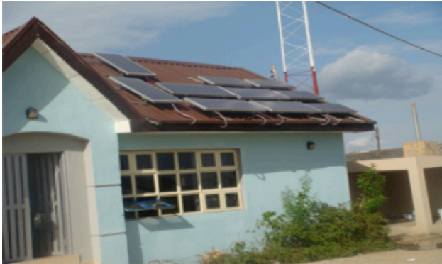
Figure 6. A picture of NIGCOMSAT Ltd Community Telecommunication Center (CTC) with Solar Panels on the Roof Top of the Center and a 200ft tower with Radio for wireless Internet Access within the community[7]
