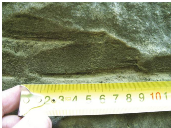
Figure 3. Traces of instruments on the portal slab
