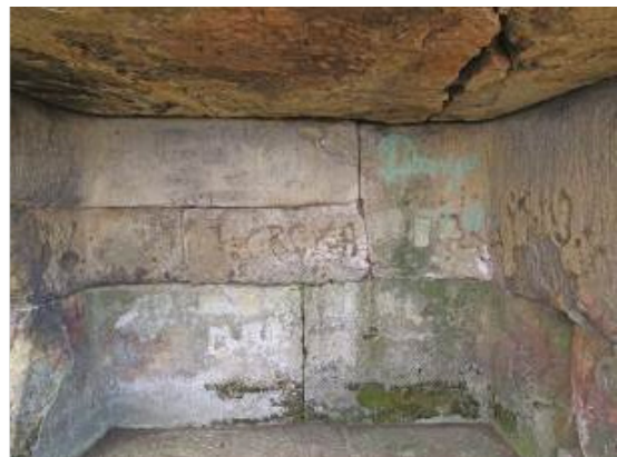
Figure 8. Polygonal masonry of the rear and side walls of the dolmen on the Mount Neksis. Ideal mating of cover and base slabs is well seen
