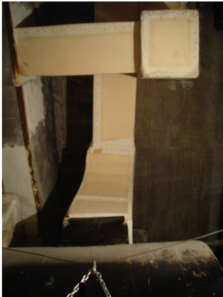
Figure 7. Outflow of air ducts of air handling unit for the main hall of the Basilica of Arantzazu
