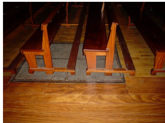
Figure 9. Return air grille of the nave
