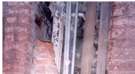
Figure 6. Damp patches can be seen near the service ducts in some buildings
