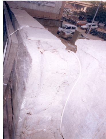
Figure 4. Splitting of coping showing the different materials. Materials with dissimilar properties are used without proper jointing detail
