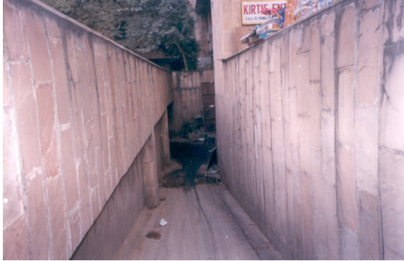
Figure 1. Discoloration of stone takes place. The stone is worn away or stained, affecting its appearance in an unacceptable way, and in some cases also affecting its damp resisting performance
