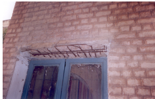
Figure 5. Deteriorated sunshade being removed from place leaving behind the exposed reinforcement. The cover for reinforcement may not have been adequately designed as per standards
