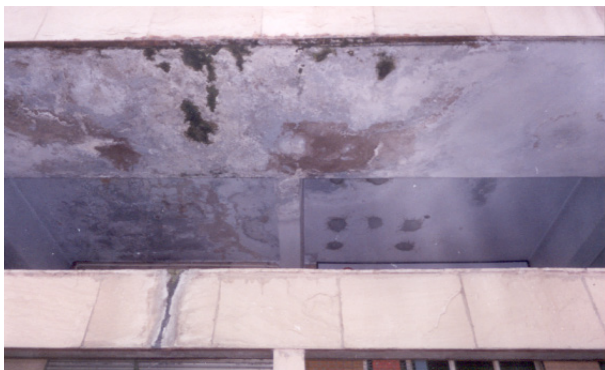
Figure 3. Seepage at the inner side of roof slab
