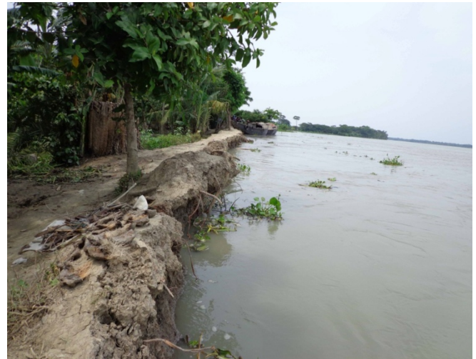
Figure 4. Faulty management of embankment and river erosion is favorable to salinity intrusion
