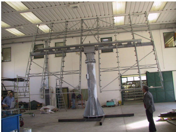
Figure 2. The PhoCUS solar tracker during the assembly process (ENEA - Galileo Avionica - ATEC Robotics collaboration). The tracking plan is of 32 m 2
