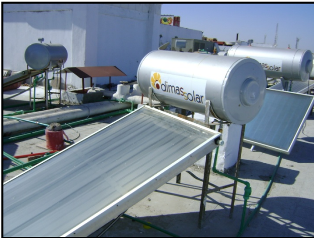
Figure 2. Solar water heater at one of the investigated four star hotels in Hurghada
