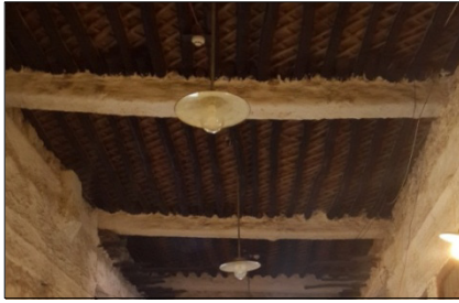
Figure 23. Traditional roof of mangrove poles (Source: authors)
