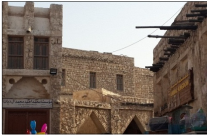
Figure 24. Traditional façade materials and the flying beams (Source: authors)
