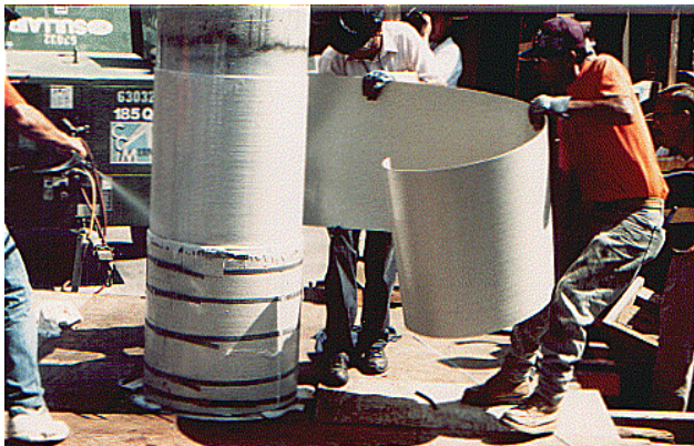
Figure 10. Installing Prefabricated Fiberglass jacket[41]
