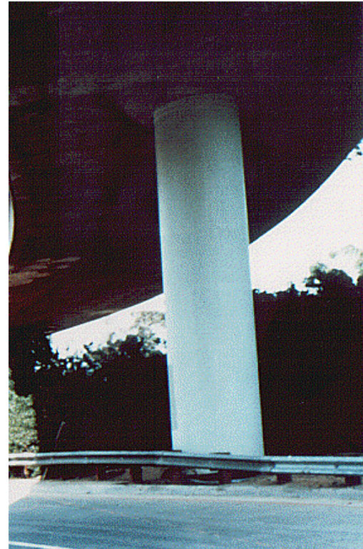
Figure 11. Snap tite applied beam surface[14]
