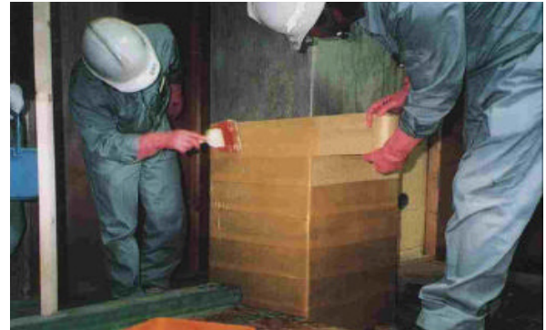
Figure 14. Attachment of Kevlar Mat with Epoxy [25,41]
