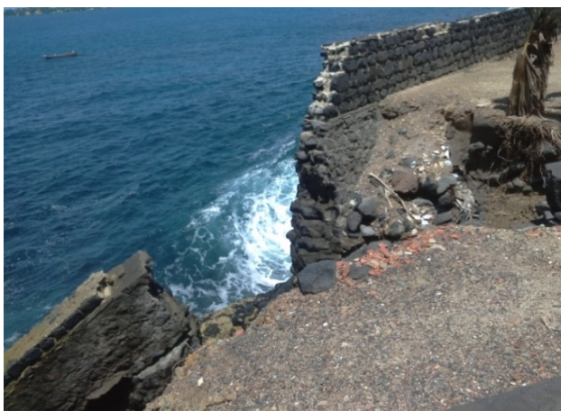
Figure 7b. Destruction by Erosion at Goree mosque
