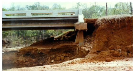
Figure 1. Observed scour beneath a bridge footing due to flooding conditions
