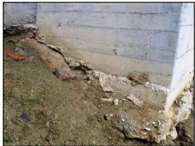
Figure 4. The endangered foundation of the building
