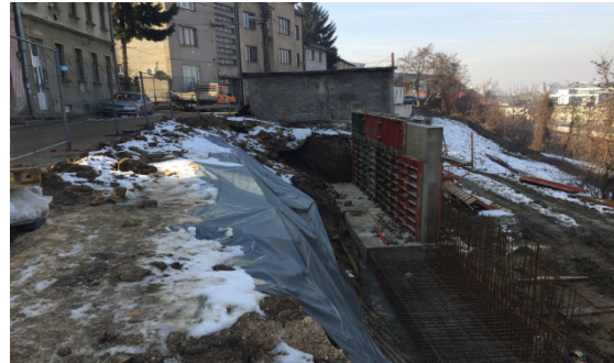
Figure 8a. Lateral spreading damage - Stolacka street in the Sarajevo Canton under reconstruction [6]
