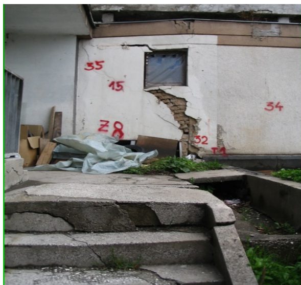
Figure 9. Cracks on the building and marks for observation Dalmatinska street in the Sarajevo Canton [1]
