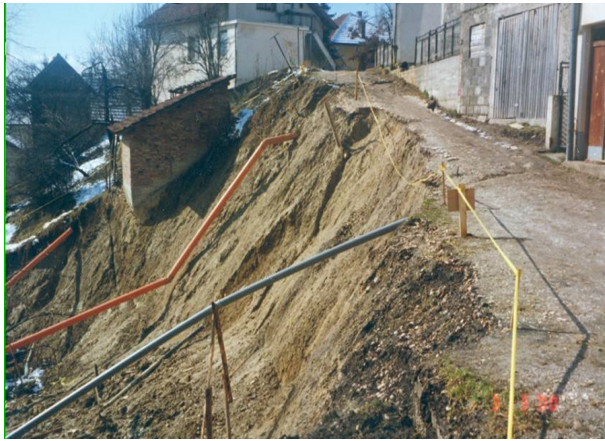
Figure 6. Consequences of landslide in the Sarajevo Canton (Kromolj), caused by rainfall, and possibly made worse by sewage leakage [5]
