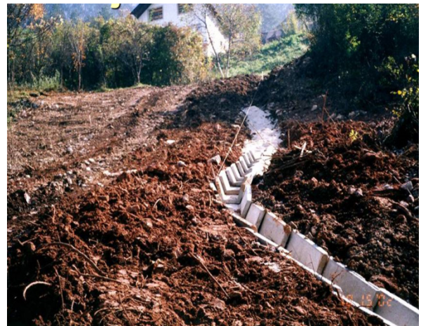
Figure 7. Illustration of the mitigation measure with open channel for surface water drainage in the Sarajevo Canton (Brusulje) [1]
