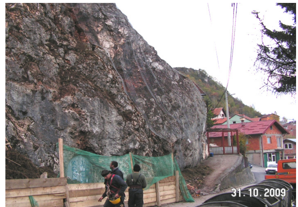
Figure 5. A rockfall/slide that occurred in Porodice Foht street in the Sarajevo Canton (2009.). with example of a rock curtain, a barrier commonly applied over hazardous rock face [1]
