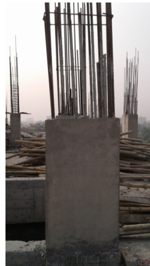
Figure 9. The clear cover is deviated due to poor workmanship and for this reason neutral axis location will be changed which must be considered in case of revised design [7]
