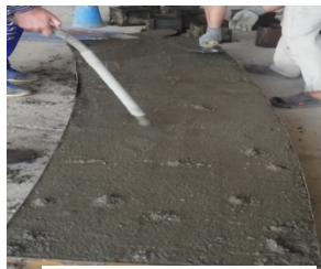
d- Casting the concrete
