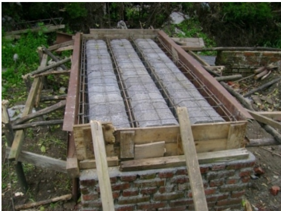
Figure 5. Placing of HCB, Reinforcement layout, Supporting System
