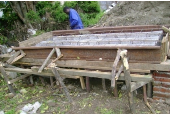
Figure 4. Formwork for ribbed-slabs
