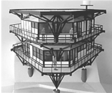
Figure 6. Tree-Shaped Timber Modular Structural System, model in 1:50 scale of a two-storey single family with 385 m 2 of construction area
