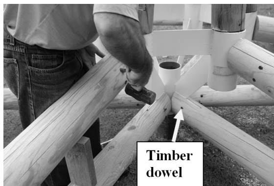
Figure 2. Fixing timber dowels
