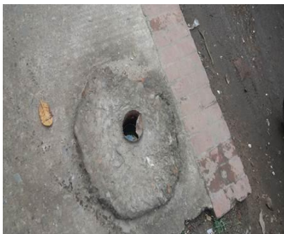
Figure 4.7. Utility Cut Holes
