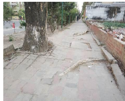
Figure 4.11. Tree Roots Damage
