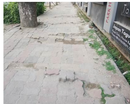
Figure 4.4. Surface Deformations
