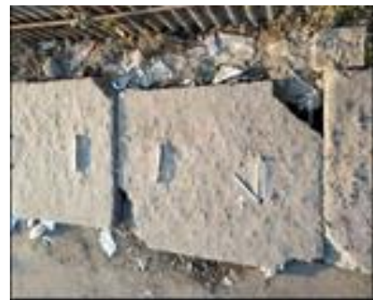
Figure 4.3. Broken Concrete Slabs
