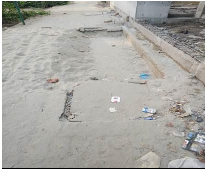
Figure 4.5. Damaged Base Layer
