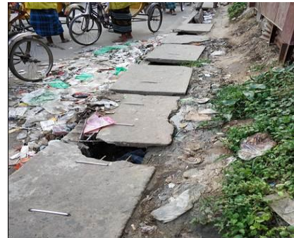
Figure 4.2. Broken Concrete Cover of Subsurface Drain
