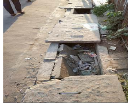
Figure 4.1. Missing Concrete cover of Subsurface Drain
