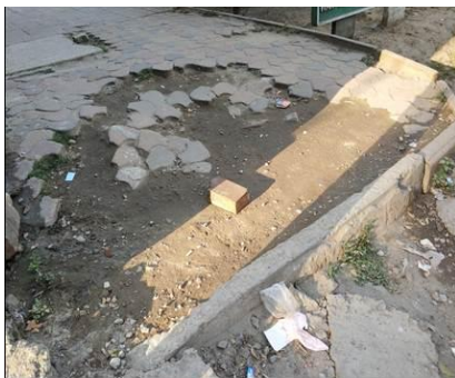
Figure 4.6. Brick or Tile missing
