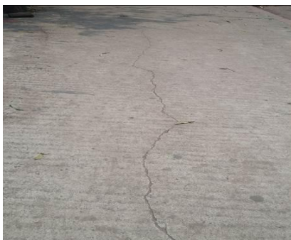
Figure 4.8. Longitudinal Crack
