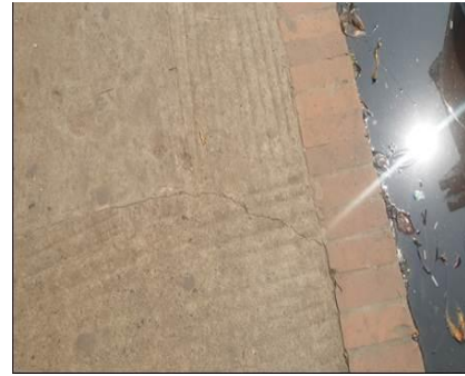
Figure 4.9. Transverse Crack
