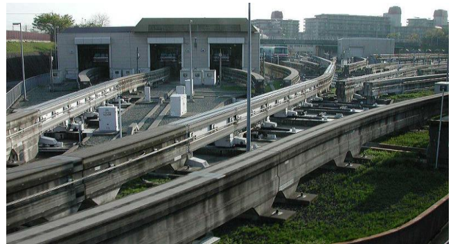
Figure 5. Example depot in Osaka, where it is possible to move the track into several branches. They move to a bright long stretches
