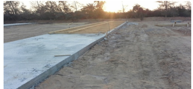
Casting bed & prepare the formwork beams (Reference: sample 30june bridges)
