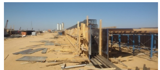
Prepare the steel works prestressed beams (sample shoubra bnha 22+400 bridge)
