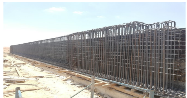
Prepare the steel works prestressed beams (sample 30june bridges & shoubra bnha)
