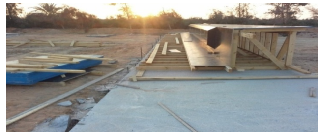
Prepare the formwork beams (Reference: sample 30june bridges)
