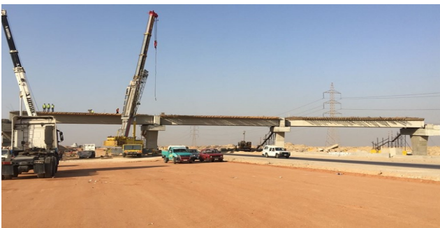
Erection beams:
