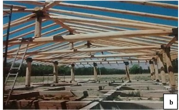
Figure 8. Multi-Purpose Centre construction details. a- excavating the foundations b- tie-beams and elevation of interior floor
