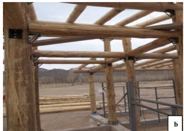
Figure 9. a- St. Andrew's cross on walls with cane struts b- Main structure with columns and wooden beams
