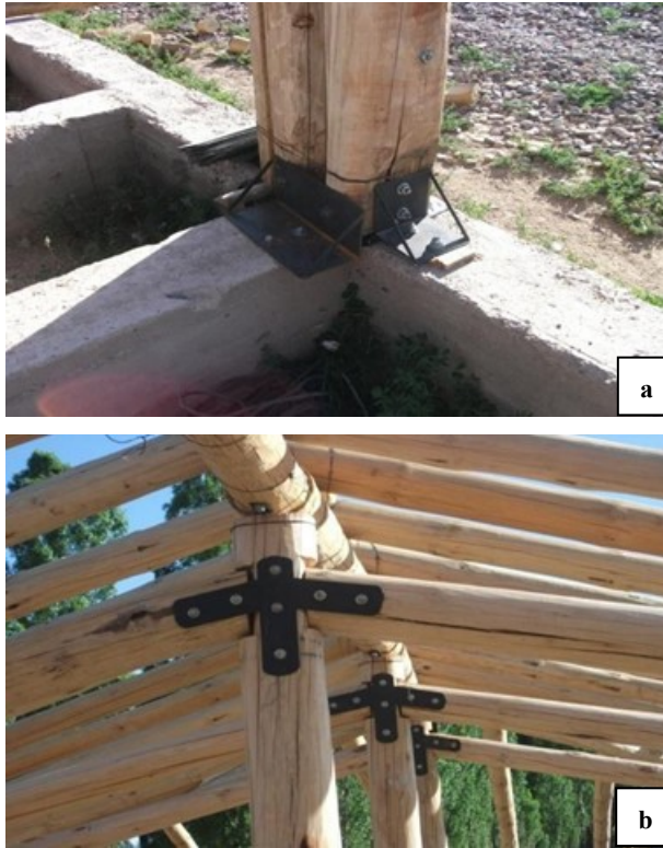
Figure 10. a- Metal plate connecting timber joints at floor level. b- Metal plate connecting timber joints at ceiling level
