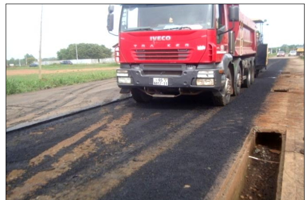
Figure 1. Binder pick-up by construction truck tyres
