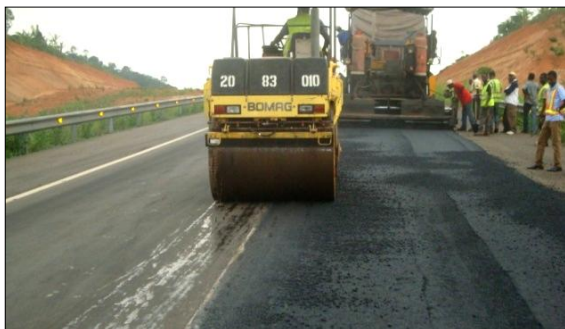
Figure 5. Compaction of longitudinal joint from cold side
