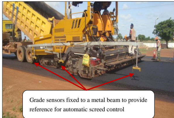
Figure 4. Use of grade sensors to provide reference for screed control
