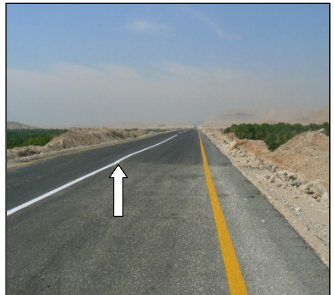
Figure 3. A heave in asphalt layer of the studied road due to swelling of an expansive soil sub-grade at El-Kawther sector, Sohag-Safaga road (Km: 1+400m)
