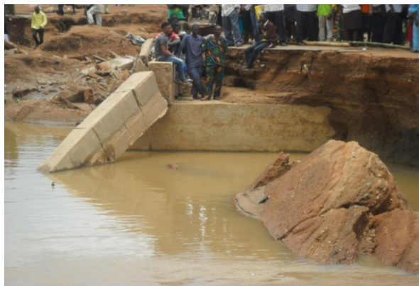
Plate 2. Collapsed Bridge during Flood event
