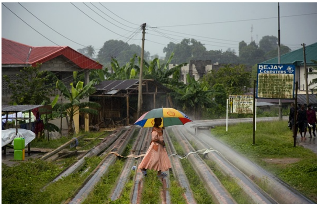
Figure 2. Erosion exposes Oil pipelines in a community of Okrika [18]
