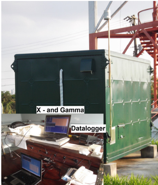
Figure 2. Trailer and instruments inside the trailer at the ACA Tower. Note the pluviometer at the top of the pole attached to the side of the container
