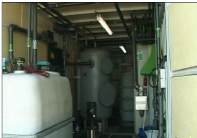
Figure 5. Container 1. Pre-filtering of the leachates
