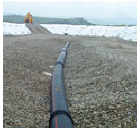
Figure 3. Construction works of the 2 nd phase at the landfill of Katerini. Leachates collection pipe. (ADT-Omega ATC, 2008)
