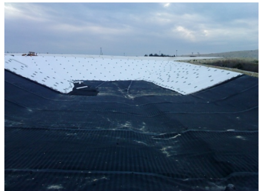
Figure 2. Construction works of the 2 nd phase at the landfill of Katerini. Artificial sealing in the 2 nd cell of the landfill. (ADT-Omega ATC, 2008)
