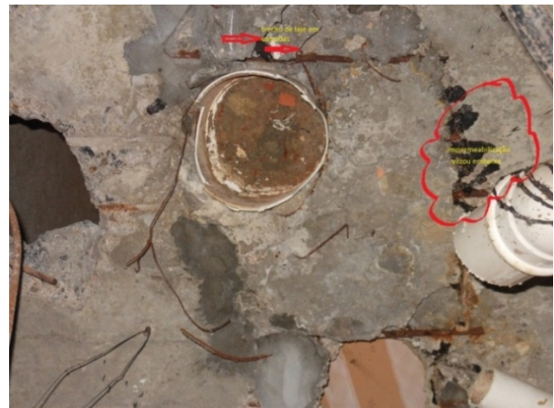
Figure 3. Top floor - slab ceiling lower-cut steel bars
