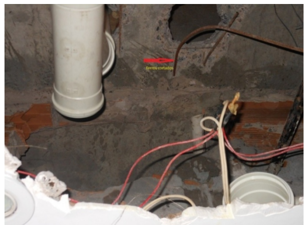
Figure 4. Top floor - slab ceiling lower - cut steel bars
