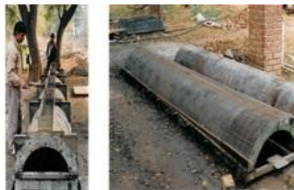
Figure 5. Prefabrication of ferrocement shell barrel vault
