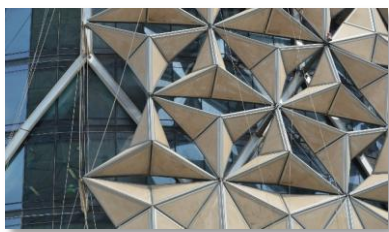
Figure 2. Dynamic semi-transparent PTFE screens of Al Bahar Tower
