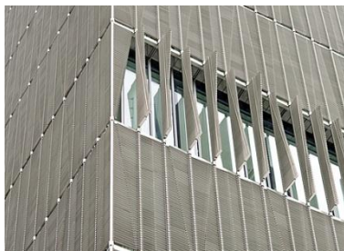
Figure 7. Perforated motorized sunshade of Q1 ThyssenKrupp
