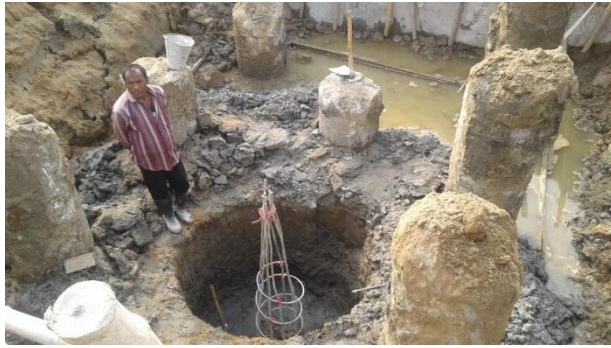
Figure 19. Pile head is not found in the specified depth [9]
