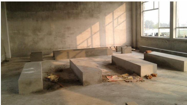
Figure 21. The author experienced in such situation of increased column load due to rearrangement of architectural plan and loading pattern after the pile construction work and rechecks the pile cap design
