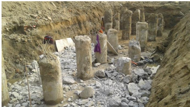
Figure 20. Pile head is not found in the specified depth which may affect the pile cap performances [9]
