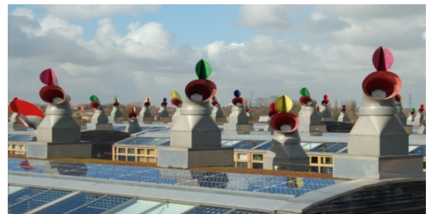
Figure 16. BedZED featuring passive ventilation chimneys, UK
