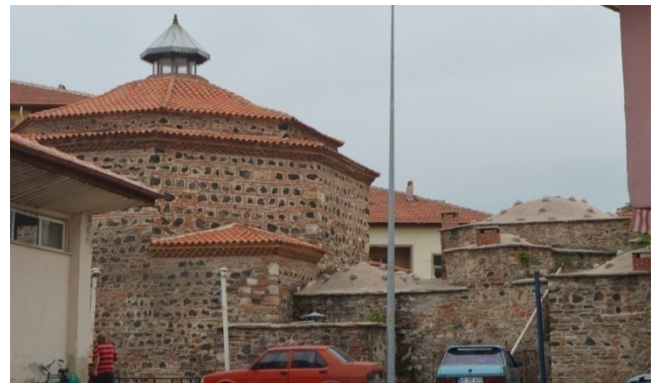
Figure 3. Wall braid in the Turkish bath with stone and brick material (Çiçin Hammam, Kula, Manisa, Turkey) [4]
