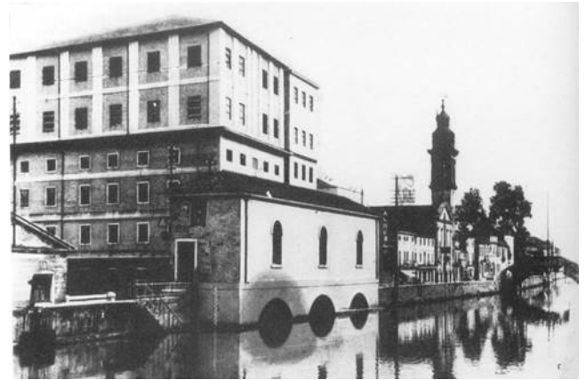
Figure 7. Old view of the hanging canal at Battaglia Terme, at the point at which the water is flowing through the Arco di Mezzo (i.e. the building with three arches in the image), originating the Vigenzzone Canal. This hydraulic device, regulating a water drop of about seven metres, was for many centuries the source of power for all the local factories
