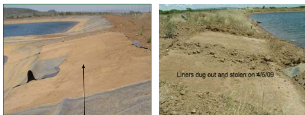
Figure 6. Stolen Plastic Carpets which is total Vandalism of Containment Dams - Source: Barrick North Mara goldmine
