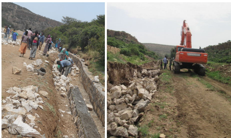
Figure 4. Mekabo scheme conveyance canal presently under construction
