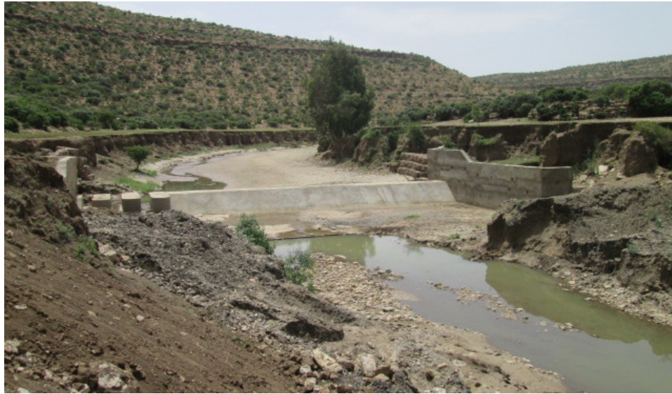
Figure 2. Constructed weir to divert water to Mekabo small-scale irrigation scheme
