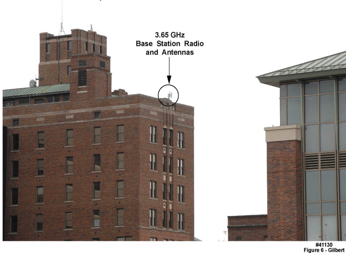
Figure 6. Franciscan Skemp medical center building in La Crosse, WI, illustrating the positioning of the three-sector 3650 MHz full duplex antenna
