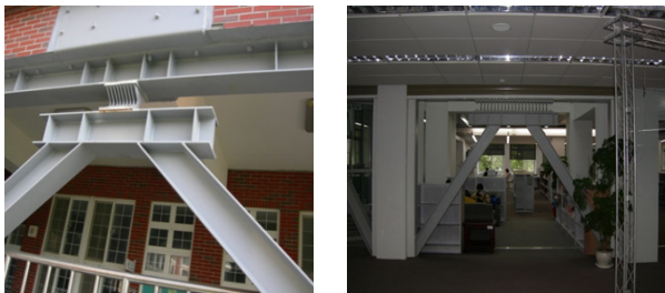
Figure 5. Two examples of strengthening building with steel yielding damper (Courtesy by Earthquake Proof System)
